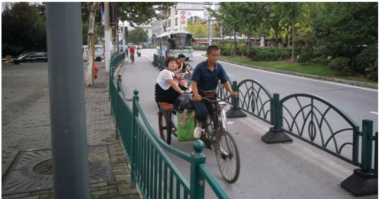
A one-way cycle track from Mexico City protects bicycles with physical barriers and markings where the barriers give way at a vehicle access point. Bottom: Cycling infrastructure seen here in Shanghai, China provides physical separation from motor vehicles through a fence. Pedestrians are also kept from entering the area.
